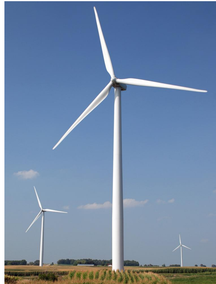
Photo by Invenergy LLC, NREL 16037
